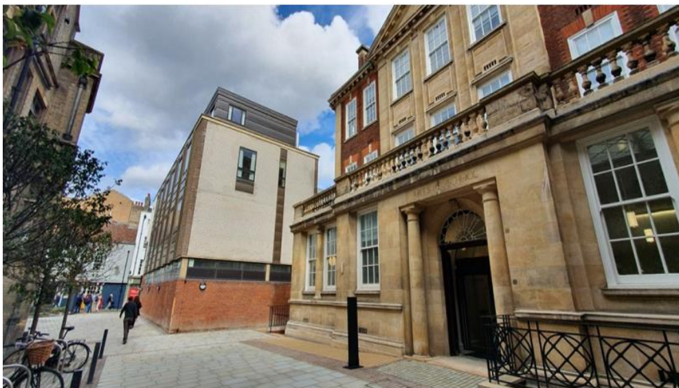
The main entrance to the ADRC and the Student Services Centre
